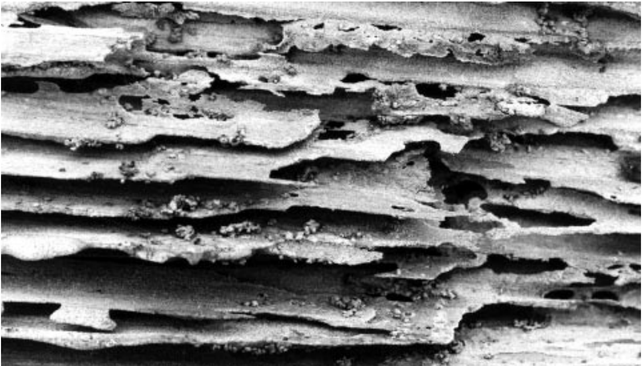
Fig. 5—Pacific dampwood termite damage. Note the loose aggregates of fecal pellets in the galleries.
