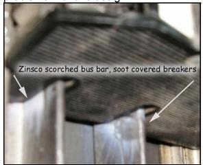
All breakers have very carefully calibrated springs and other components. Arcing where these breakers contact the bus bar is a common problem with this design. This can result in the overheating and incapacitation of the breakers. We have seen these breakers with their cases blown out and leaving soot on the inside of the enclosures.
