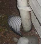
Gutter mounts failing and the downspout is disconnected. Keep downspout drains clear of mulch and debris.
