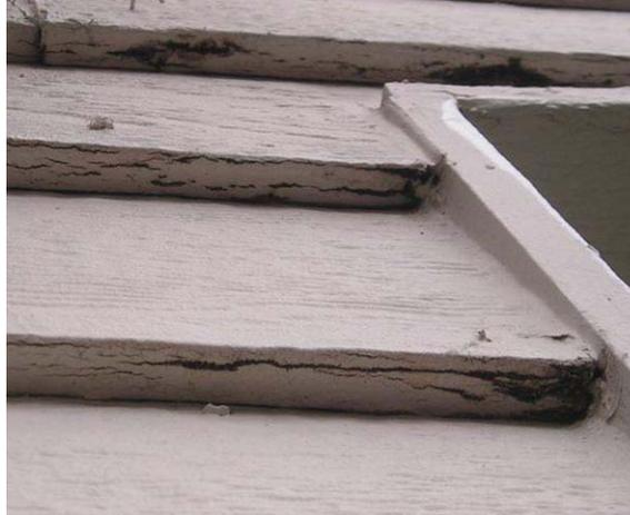
The bottom edge of LP lap siding is where the failure is first evident.
