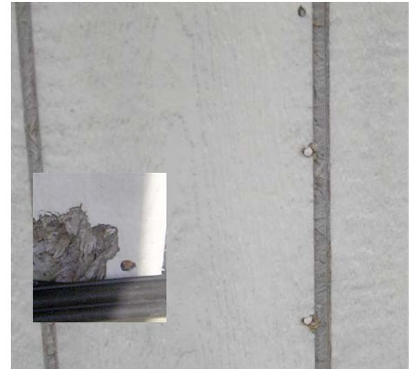
Sheet LP fails in the grooves, nail holes and penetrations.
