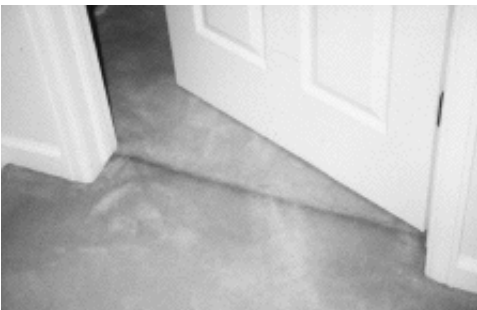
An example of impaction. Supply air registers located inside this bedroom pressurize the room. The air in the positively pressurized bedroom seeks the path of least resistance toward the lower pressure of the main body of the house, where the cold-air return is located. Air passes underneath the closed door, causing the carpet to act as a filter for particles. Over a period of time, the carpeting will pick up enough airborne particles to cause the discoloration.
