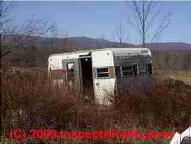
**Trailer** traditionally describes a usually small, wheeled, home with a history and image of flimsy construction such as wooden 1x3 wall framing clad with aluminum siding, virtually no insulation, and low quality leaky windows.
